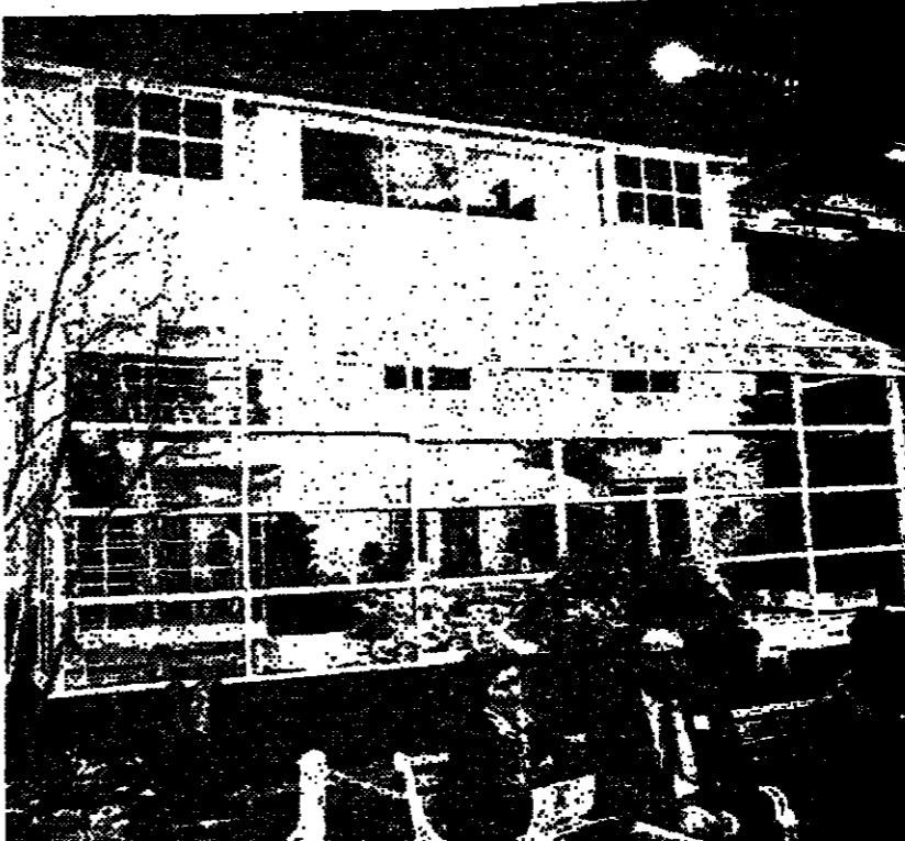
The huge glass conservatory of Future House 2000 is designed to trap the sun to provide solar energy for the house
